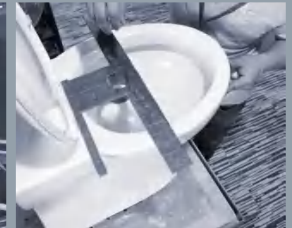
6.QC:Cover Testing Air Testing Cleaning & Water Teting Customers Testing.
